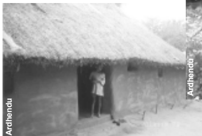
Straw as roof material
