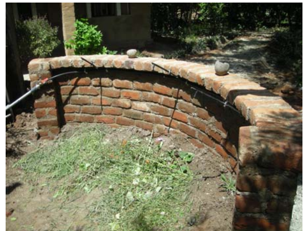
Washing area constructed with provision for mulching, use of sprinkler pipes for taps
